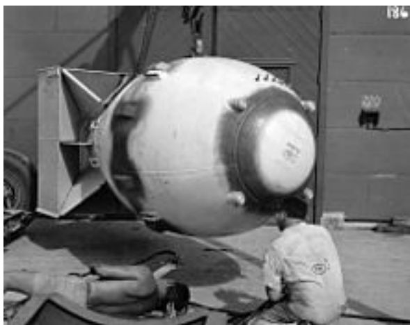
The team readies the Fat Man bomb, sprayed with liquid sealant on the casing's seams, on one of the Northern Mariana Islands, Tinian.
